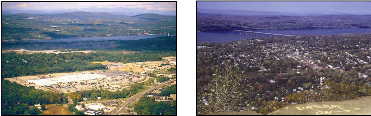
Figure 9.1. Two contrasting development models: single-use, auto-dependent commercial strip displaces nature along Route 9, or a mixed-use, walkable center embedded in nature, like the City of Beacon.
